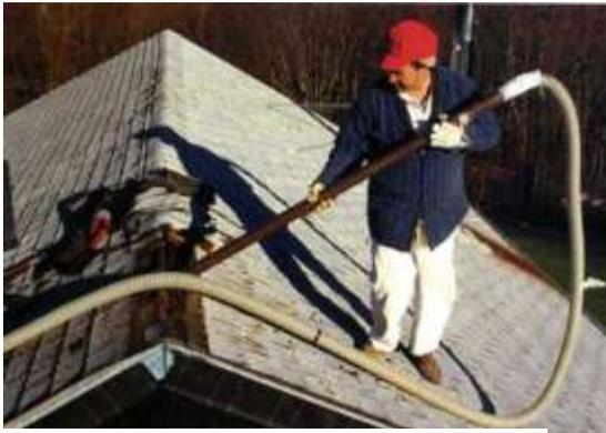
**Figure 3:** Installing attic insulation from the roof.
